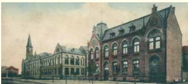
Dobový pohled na budovu radnice i školy. Dnes v obou budovách sídlí úředníci. Period view on the Town Hall building and school herewith. Today, both buildings serve to officials.
